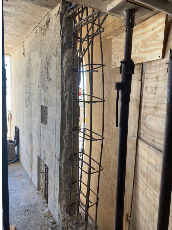
Picture 1: Concrete repair on walls in garage
