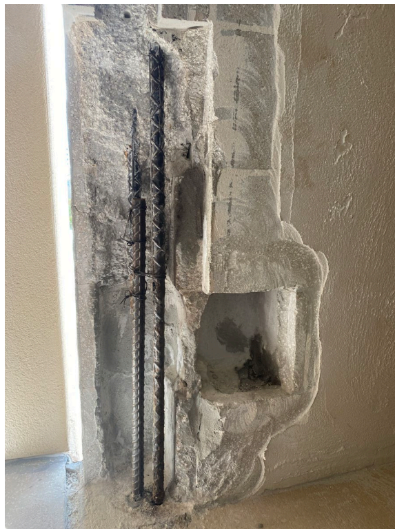
Picture 4: 4 th floor stairwell jamb repair
