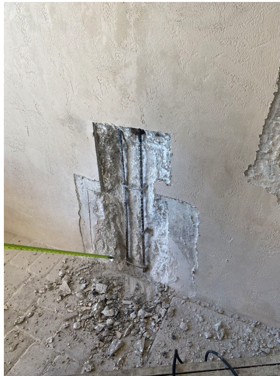
Picture 2: Concrete repair on walls in garage
