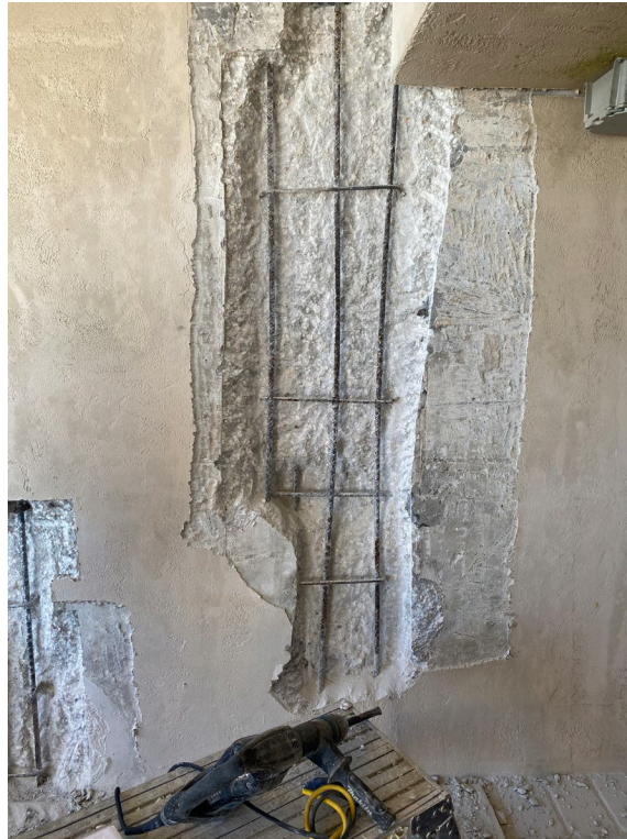
Picture 3: Concrete repair on walls in garage
